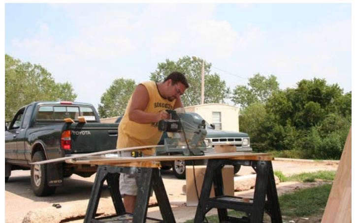
Colin Miles working on some of the construction of the dorm.
